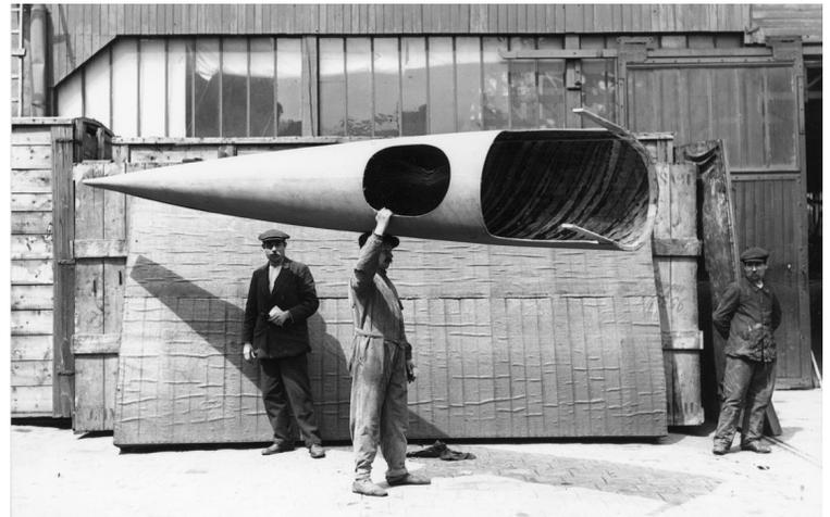
Workman carrying a complete Deperdussin monocoque fuselage, Deperdussin factory, Paris, about 1912
